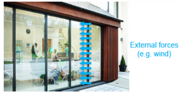
Figure 12: External forces acting on the glass panel.
